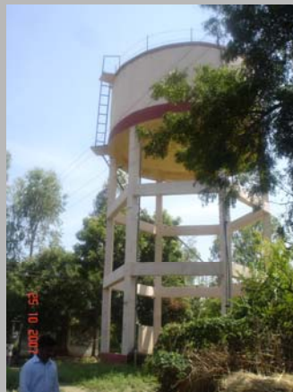
A water tank. The project that marked the beginning of a new era for Gangadevipalli
